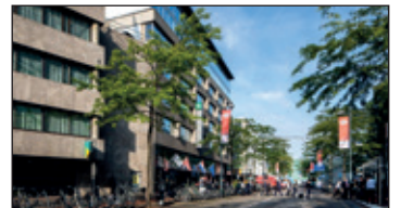
HAMPSHIRE HOTEL CROWN EINDHOVEN Vestdijk 14-16 - 5611 CC, Eindhoven
