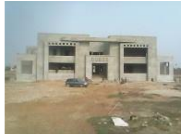
Goal project buildings (from top) Jacobabad, Abbottabad and Sukkur.–Via PFF/June 12
